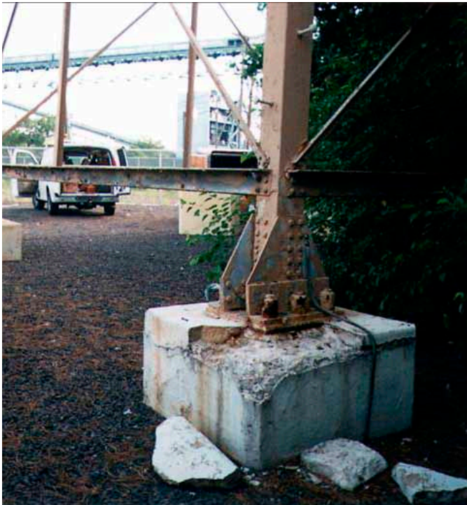
Severe damage to concrete foundation
