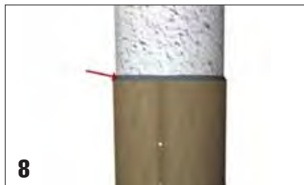
8 Install FX-763 Hydro-Ester® Low-Modulus Trowel Grade Epoxy at the head of the jacket and finish to a 45° tapered bevel, creating a water- and chemical-resistant barrier to the repair system.
