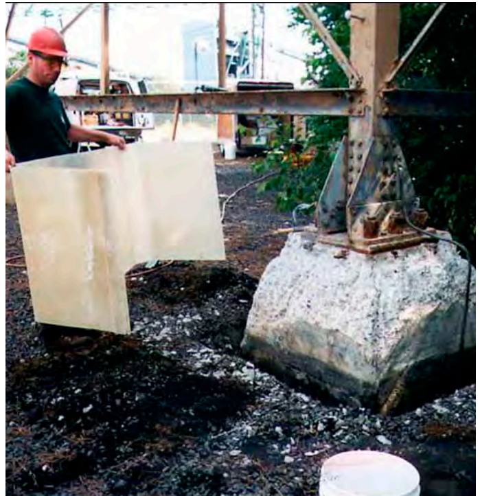
Foundation prepared and excavated; FX-70 jacket installed below ground level for additional protection
