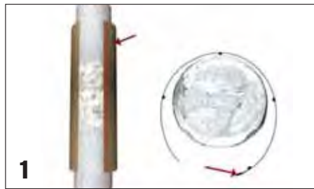
1 Install a bead of FX-763 Hydro-Ester® Low-Modulus Trowel Grade Epoxy into the locking groove of the jacket and place FX-70 jacket around the pile to be repaired.
