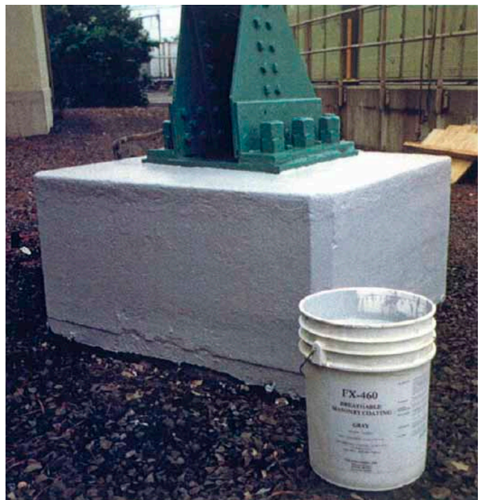
FX-70-6 Hydro-Ester® Multi-Purpose Marine Epoxy Grout used as bottom and top seal, FX-928® Concrete Mix used to restore structural capacity of foundation
