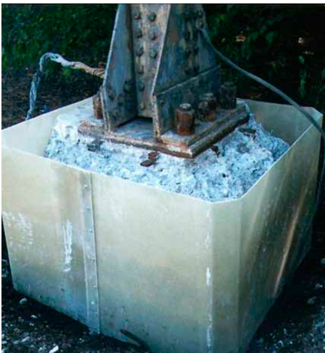
FX-70 jacket installed and backfilled
