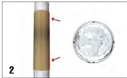
2 “Close” the jacket by inserting the tongue into the locking groove of the jacket. Position the jacket so there is 18–24” of undamaged pile inside the jacket above and below the damaged area.
