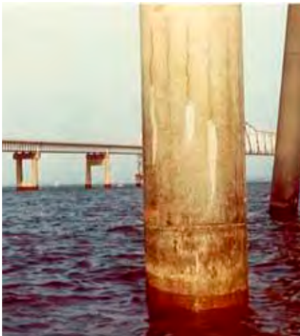
▲ Example of pile "scour"
