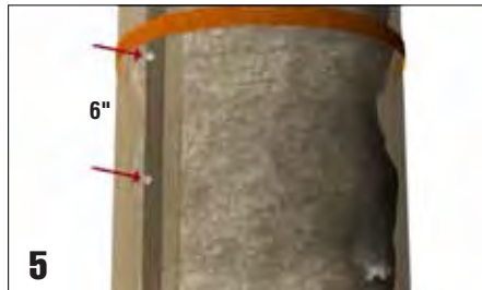
5 Install a stainless steel, self-tapping machine screw every 6” o.c. to secure the tongue-and-groove joint.
