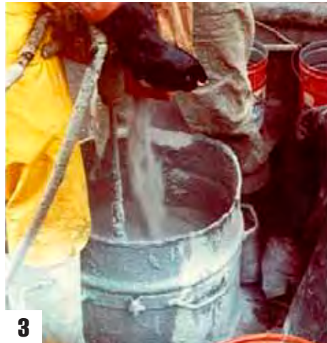
3 ▲ FX-70-6 grout mixed in work boat
