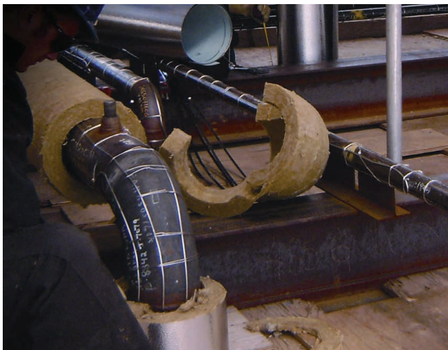
ProRox PS 960 NA is fire resistant and water repellent that saves energy, while also providing optimal protection for personnel and equipment.
