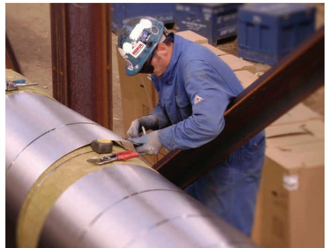
ProRox PS 960 NA requires nothing more than a serrated knife for precise cuts that can be made quickly and easily at the point of installation, reducing waste and manpower hours.
