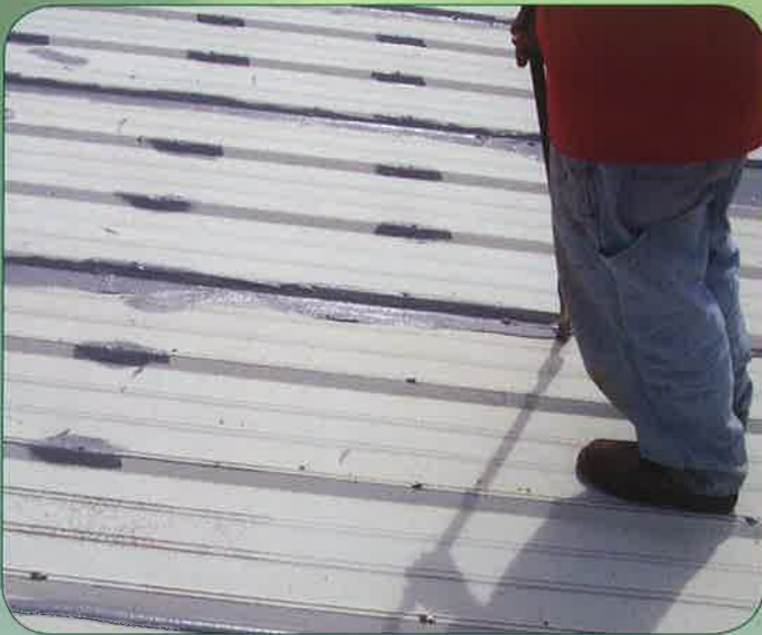
HER seals seams and fasteners on metal roofs. FLUID APPLIED AND NO FABRIC.
