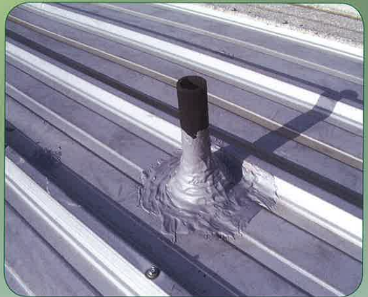
HER can easily seal flashings and roof penetrations.
